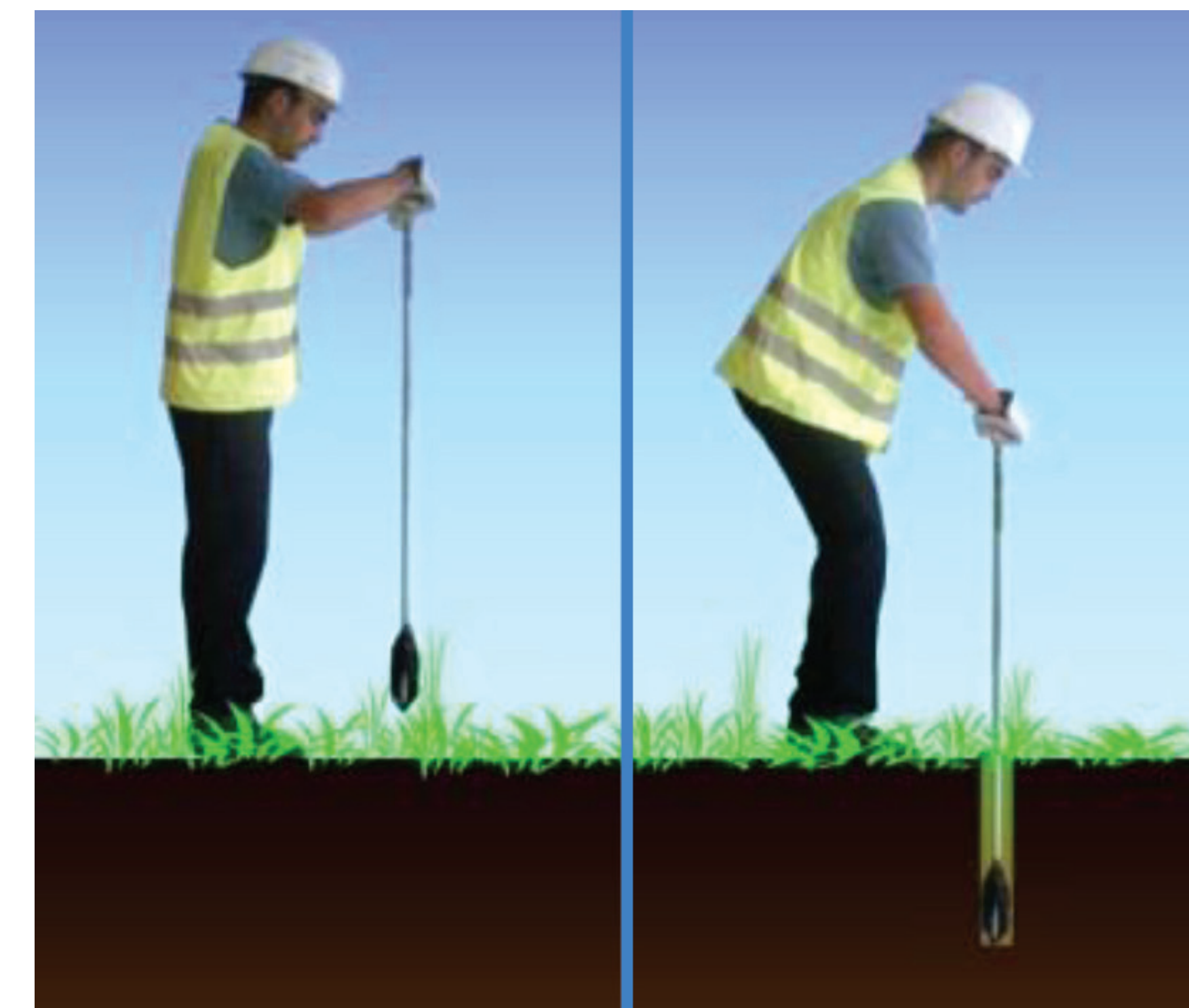
Installation of a Source Area or Near-Slab Soil Vapor Well
