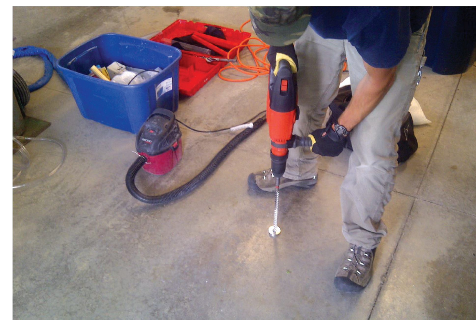
Installation of a Sub-Slab Soil Vapor Pin
